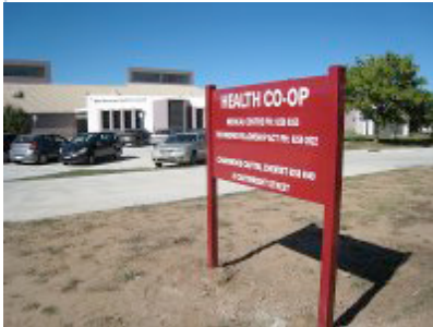
West Belconnen Health Centre
